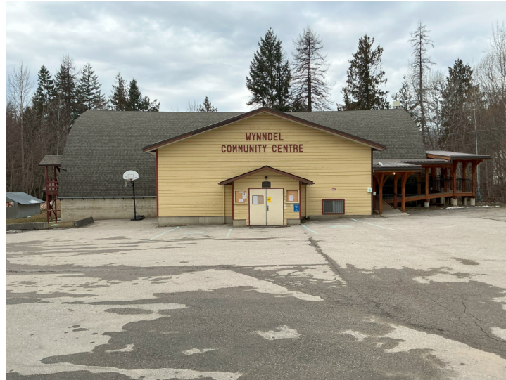
Photograph 1: Exterior east elevation view
