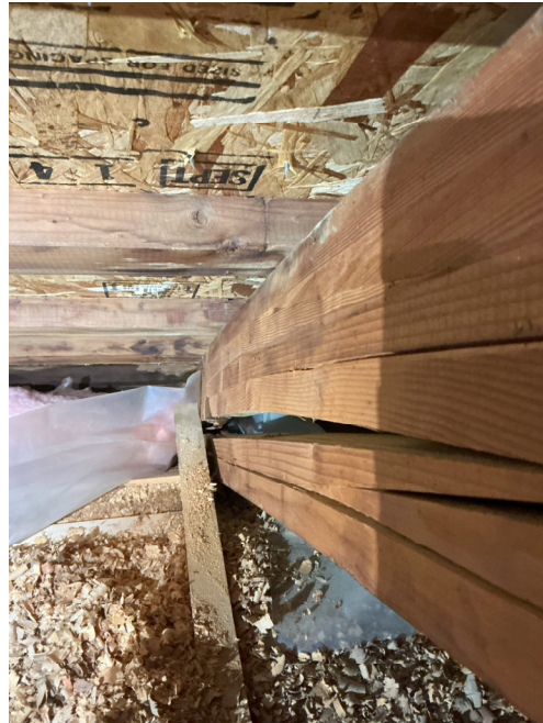
Photograph 3: Cracked / delaminated arch
